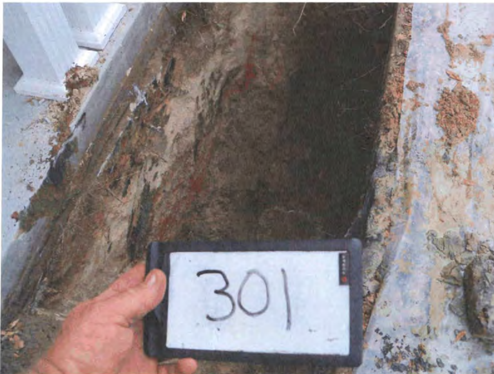
Picture 2: UST 301Ash excavation pit.
